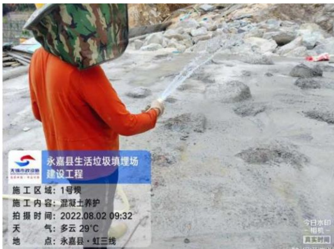
施工期洒水抑尘
